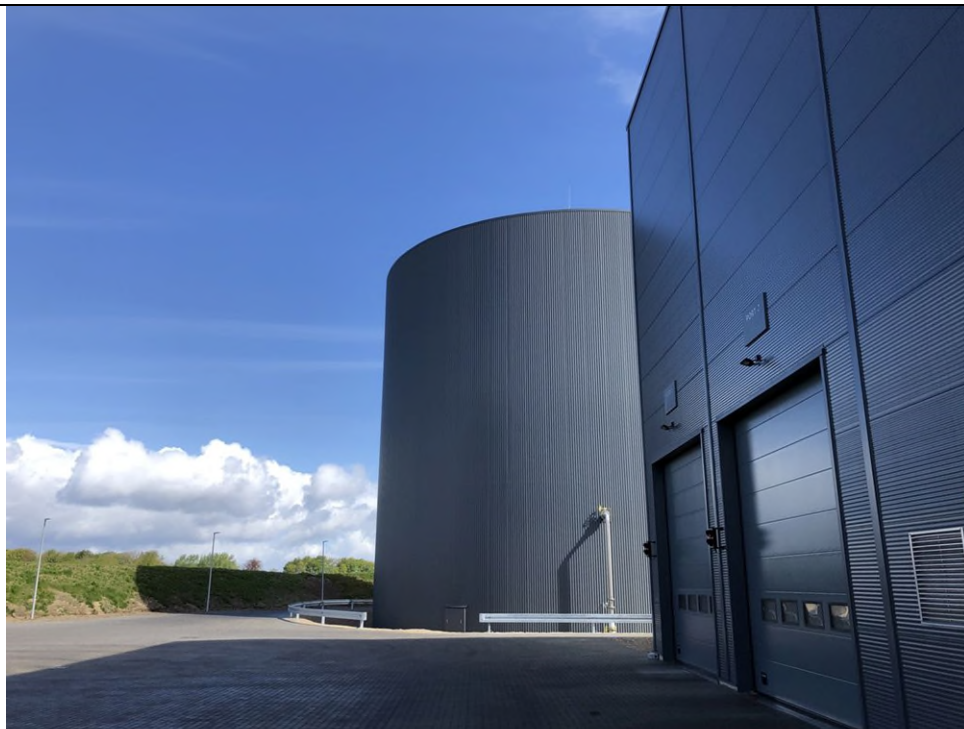
Figure 6: Biogas plant in Videbæk. Manure becomes biogas, renewable energy supplied to the local district heating.
